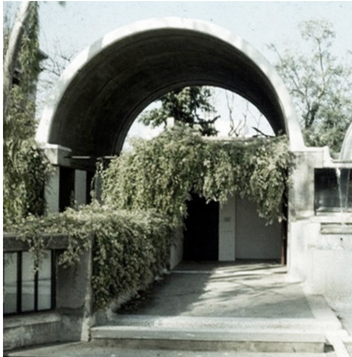
(Figure 25) Sangath's Dome roof structure
