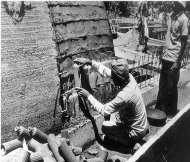
(Figure 20) Concrete shells were handcrafted
